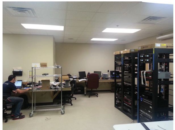
M3 staging facilities are used for system pre-fabrication and testing
